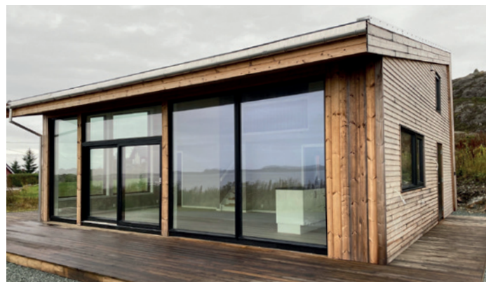
SLIDING DOOR, FIXED FRAME AND TOP SWING WINDOWS IN KOPERVIK, ON KARMØY
